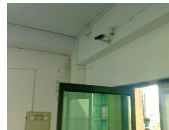
Fig. 12 (b). Right Side view of CCTV Camera Setup
