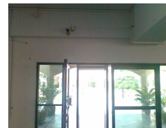
Fig. 12 (c). Front view of CCTV Camera Setup
