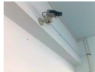
Fig. 12(a). Left Side view of CCTV Camera Setup
