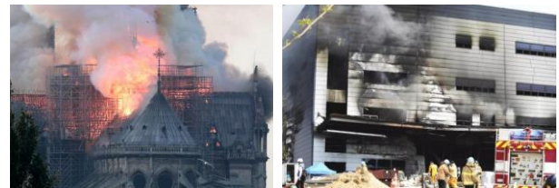
Fig. 1. The fire situation.
