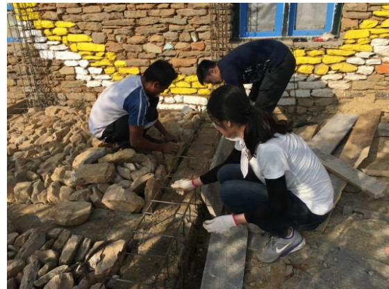
Fig. 8. Toilet design and (partial) construction by student groups.
