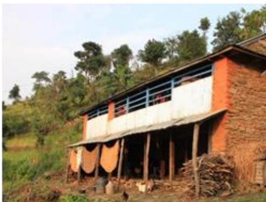
Fig. 3. Local village house before the earthquake.
