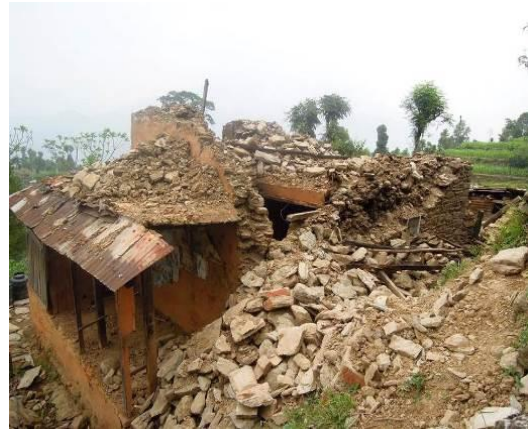
Fig. 4. Local village house after the earthquake.
